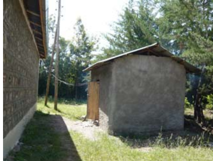
New Back-up Generator House
