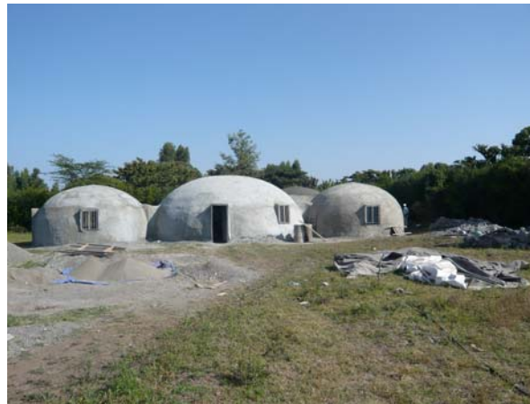
Guest House Under Construction
